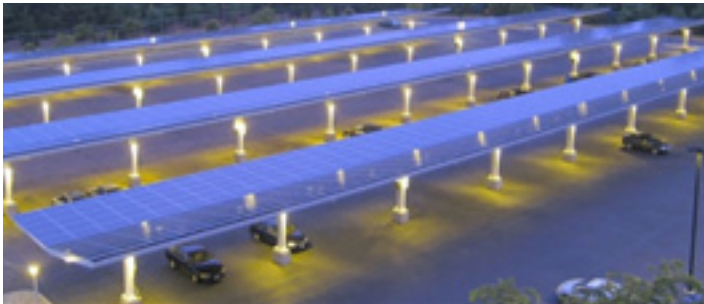
Figure 53: Solaire Generation Solar Canopy Design Source: http://www.solairegeneration.com/
