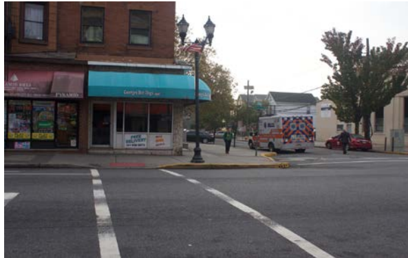
3. Reverse bump encourages longer crosswalks, no pedestrian countdown signal.
