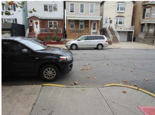
7. Missing crosswalk and truncated dome on Prospect Ave. and E.27th street.
