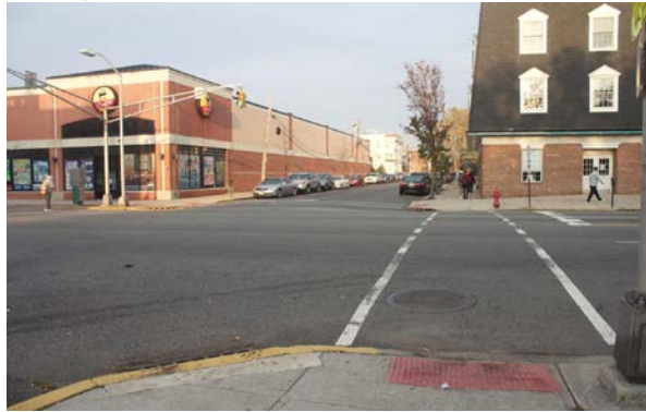
1. Long crosswalk, missing truncated dome, no pedestrian countdown signal.
