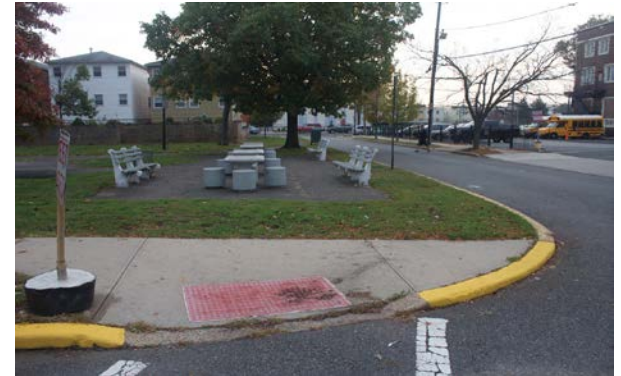
4. Park in front of school missing sidewalk.
