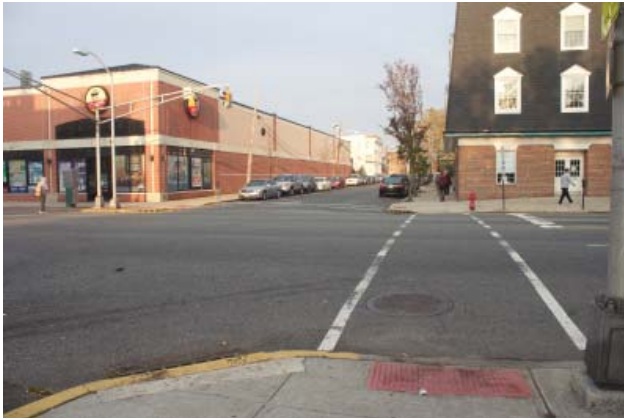
Figure 34. Before: Existing intersection
