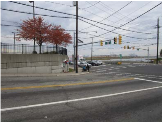
Figure 36. Before: Existing crosswalk
