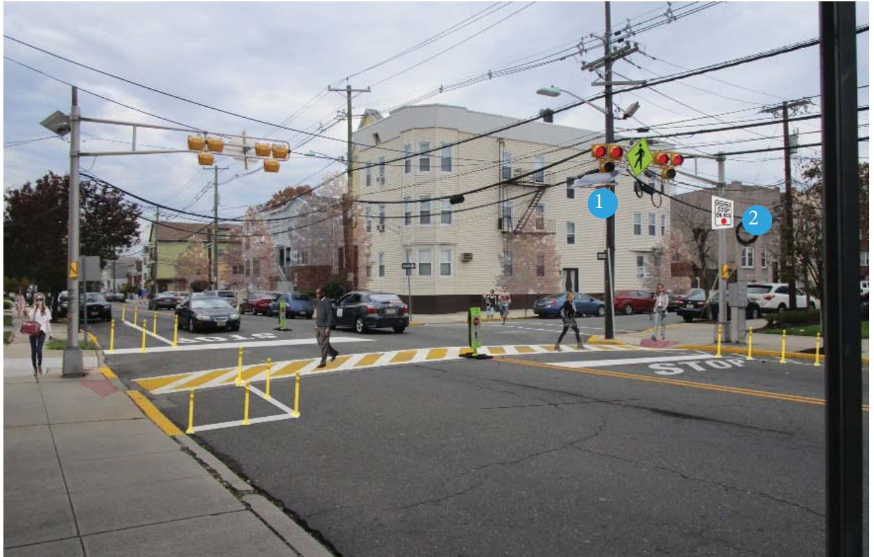
Figure 29. After: More visible pedestrian signage
