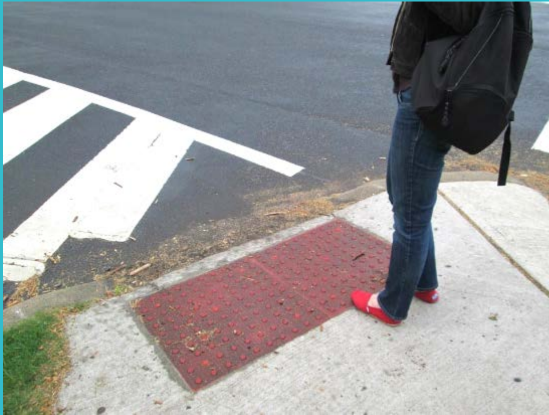
Photo: NJ Safe Routes to School Resource Center
