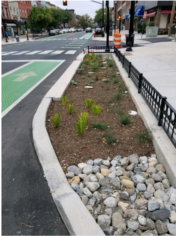
Figure 71: Bioswale at the curbside
