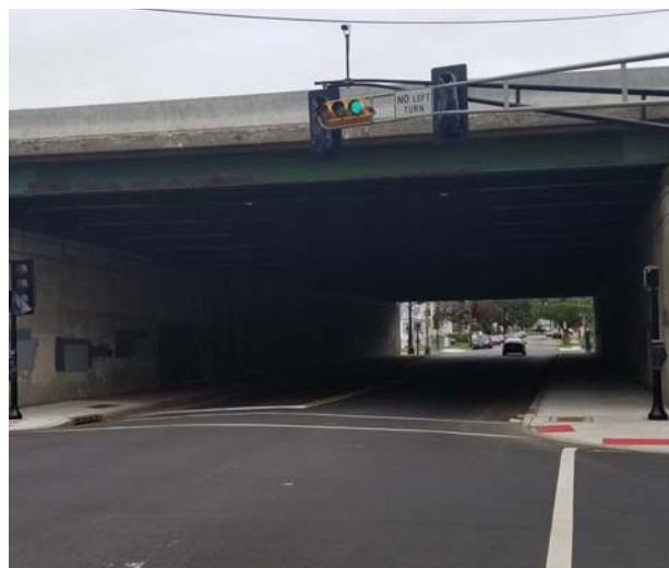
Figure 58: Image of the underpass below the Parkway
