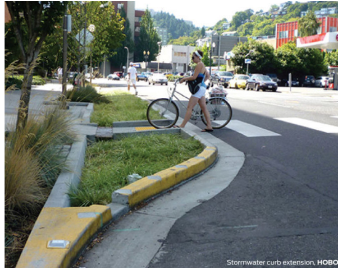
Fig.24. Curb Extension with Infiltration Planting Credit: NACTO
