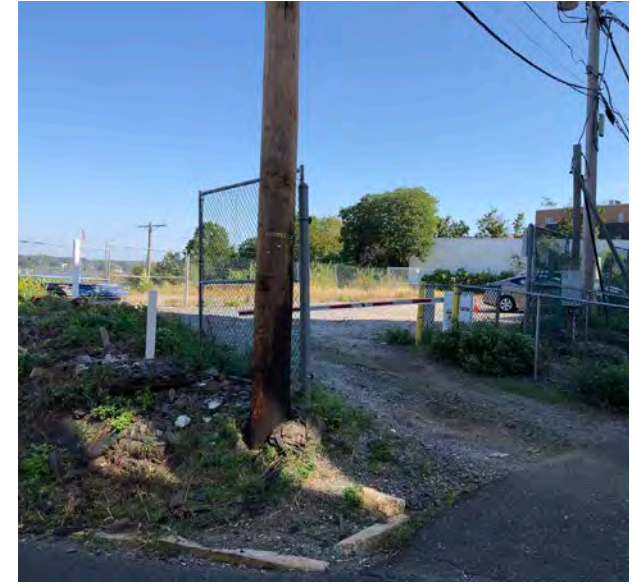
Contaminated site at 24 West Front Street
