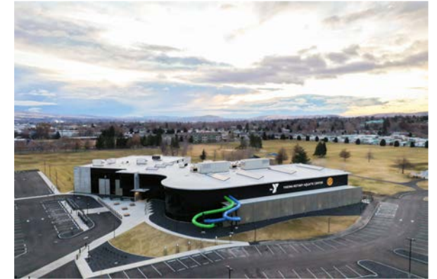
YMCA and Yakima Rotary Aquatic Center- Yakima, WA
