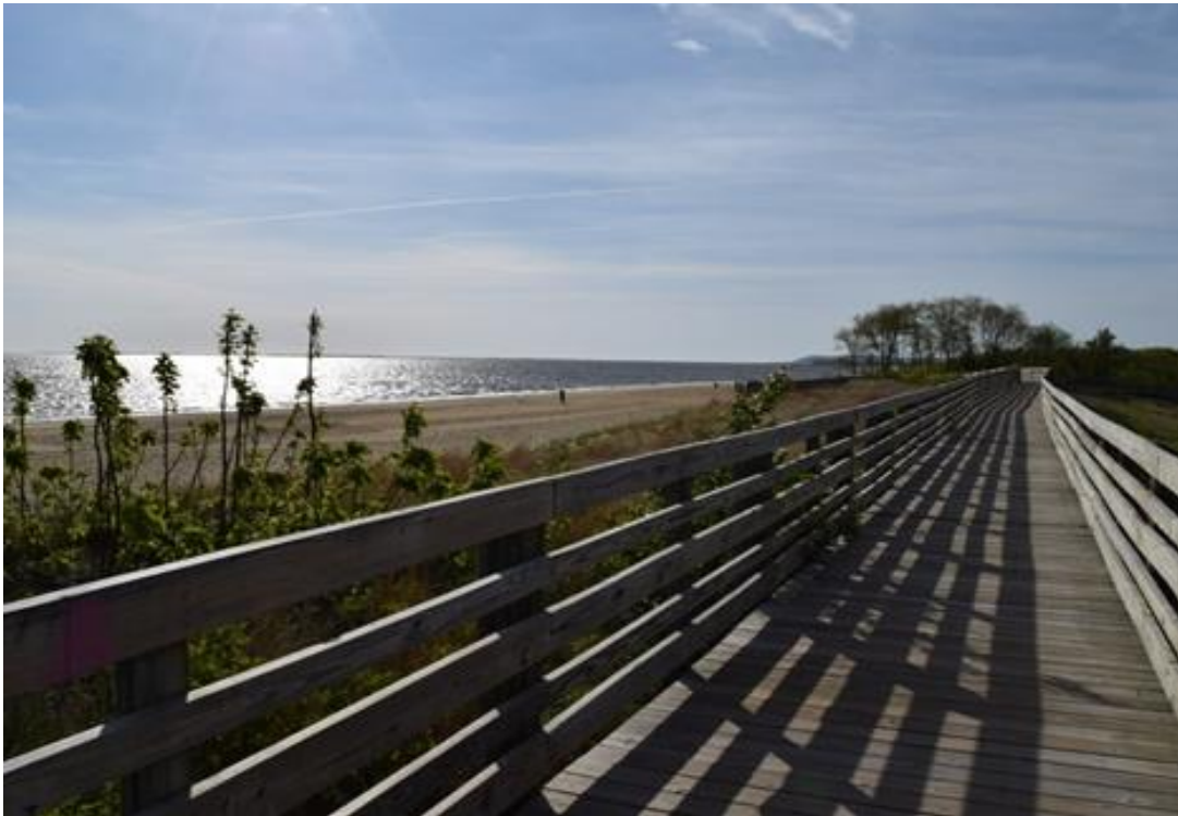
Figure 10. Restored Baywalk in Keansburg (Baldwin 2020)
