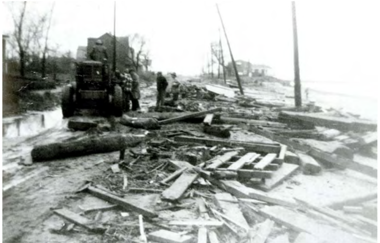
Damaged infrastructure in Union Beach following a storm in the 1900s
