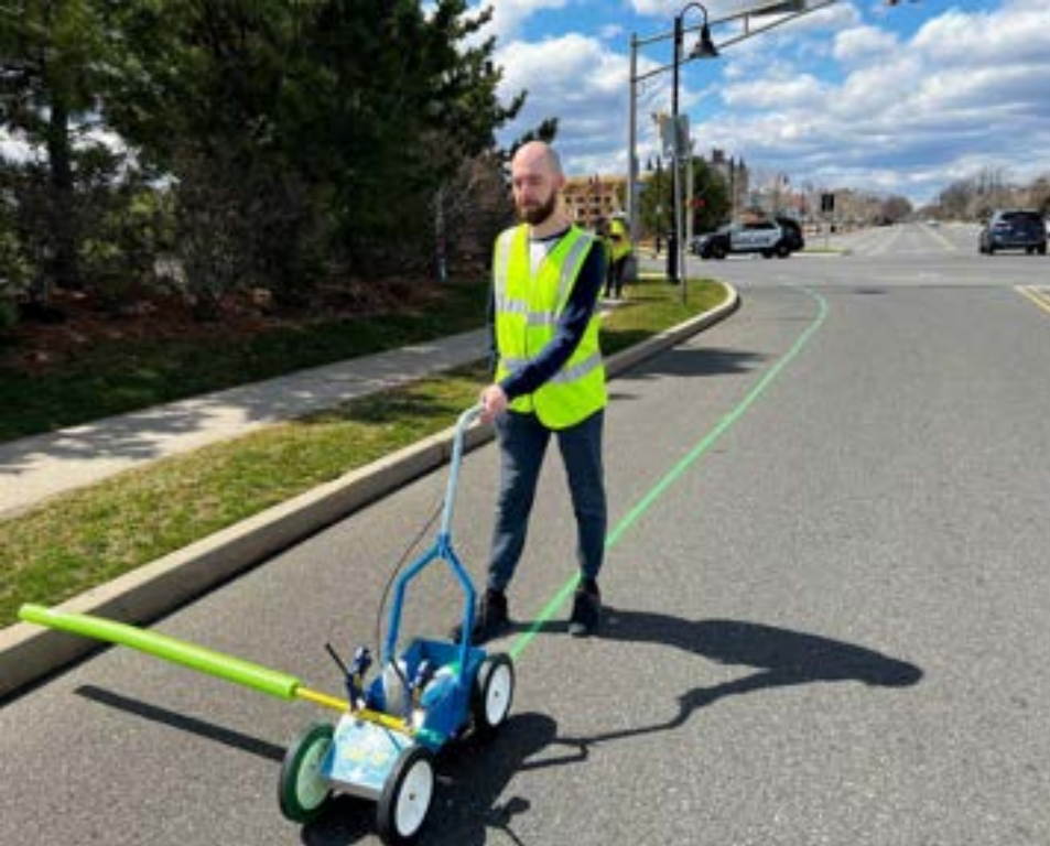
Striping the bike and scooter lane
