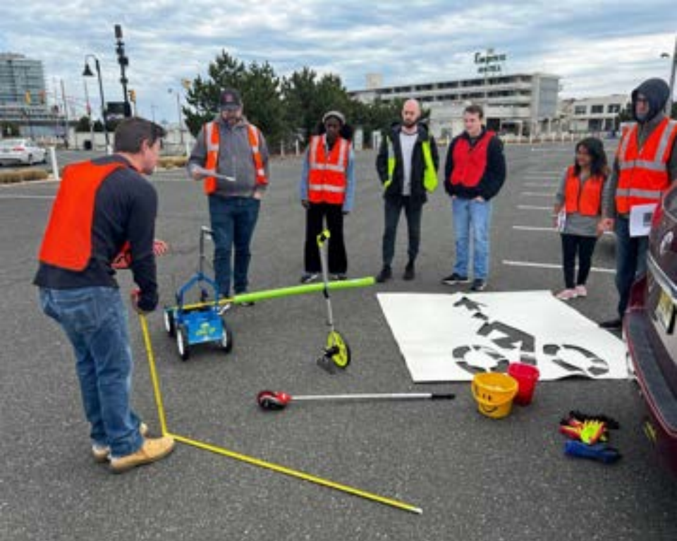
Planning the day's work (left) and measuring out and marking where the bike and scooter lane would be striped (right)
