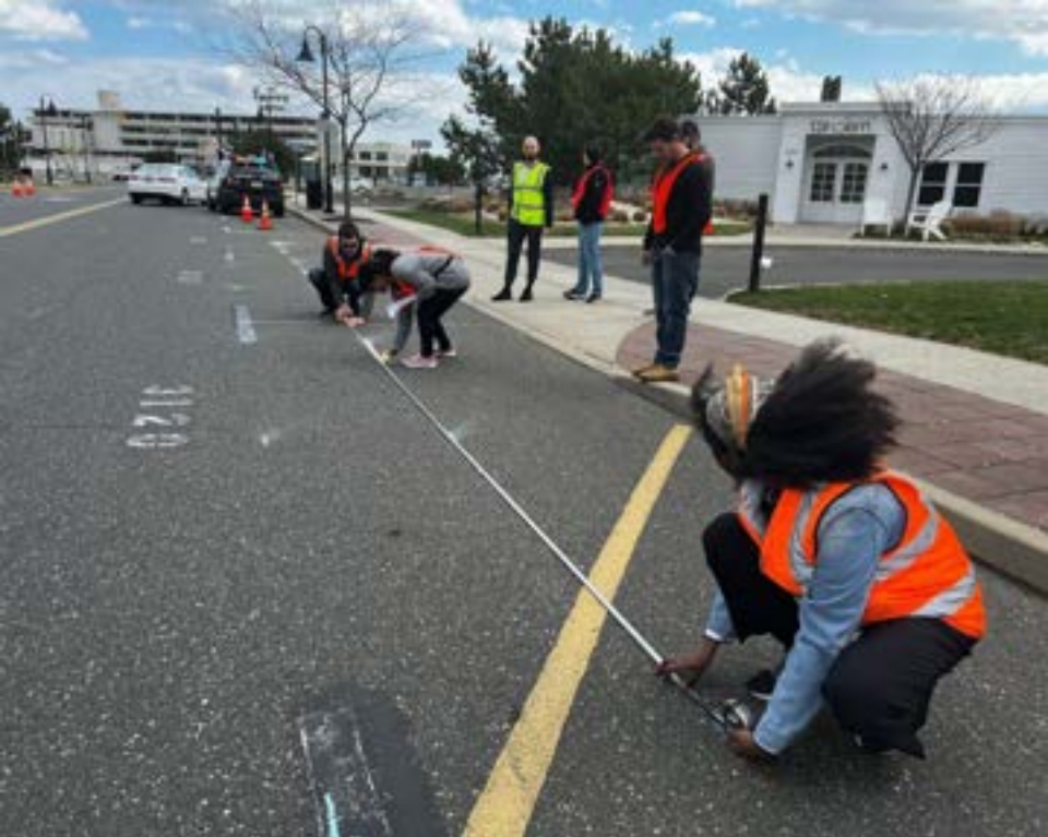
Planning the day's work (left) and measuring out and marking where the bike and scooter lane would be striped (right)
