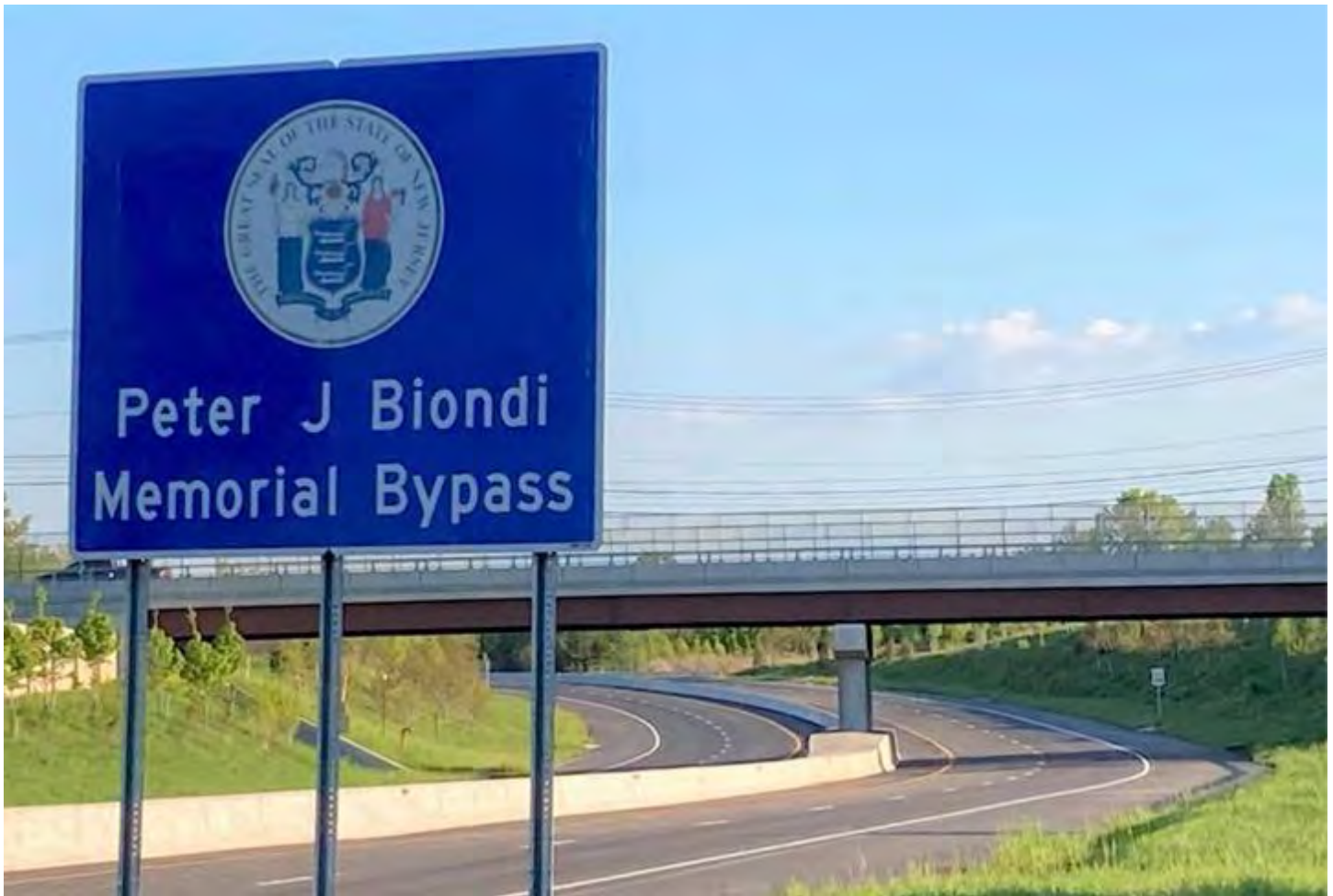
The recently complete Route 206 Bypass (Source: TapInfo )
